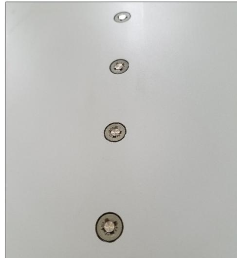
Figure 6. Blind fasteners installed and shaved flush with the OML
